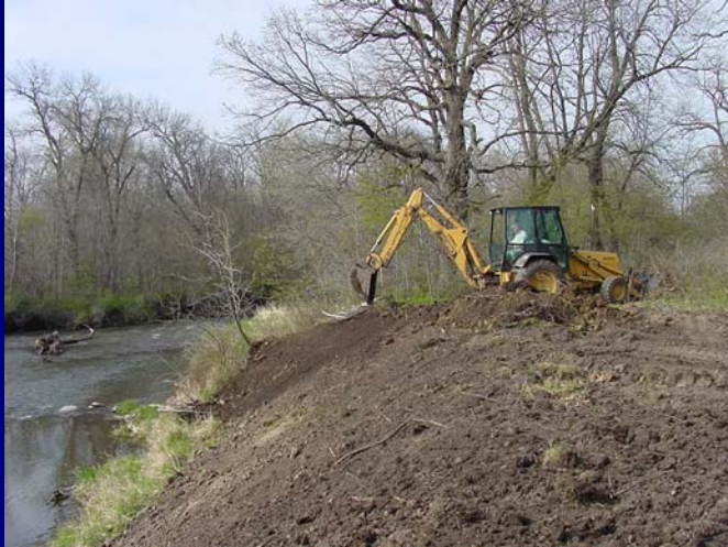
Excavating to a 2:1 Slope
