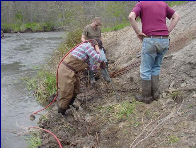
Jetting holes for willow sprigs
